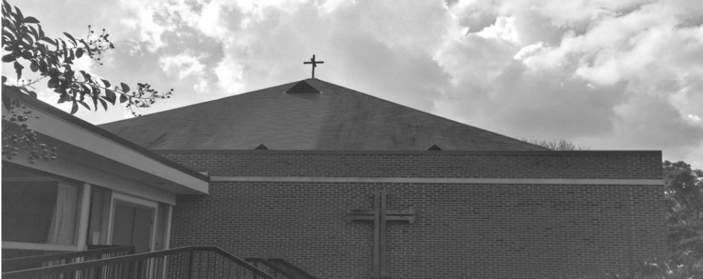
Sanctuary Steeple Cross
