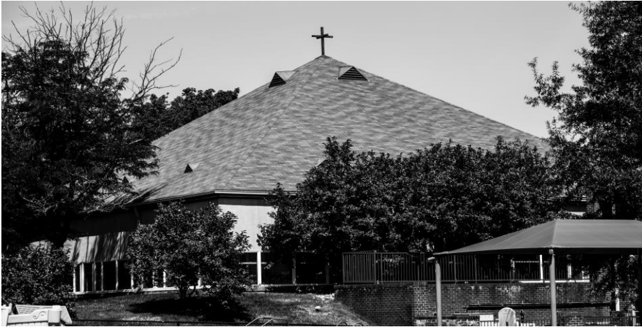
Sanctuary view from Rear Parking lot
