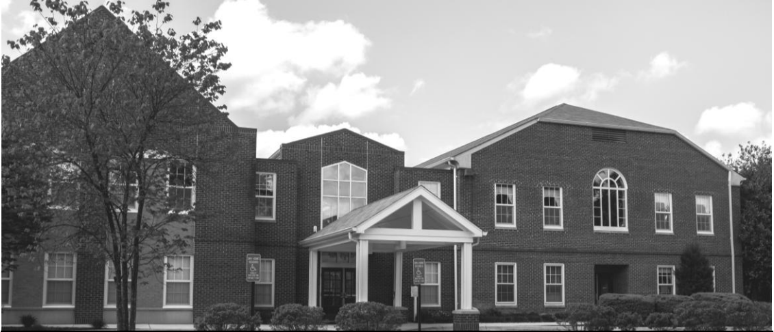
Spring Street Facing Entrance
